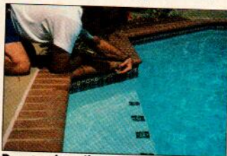
Dye-testing tile cracks.
